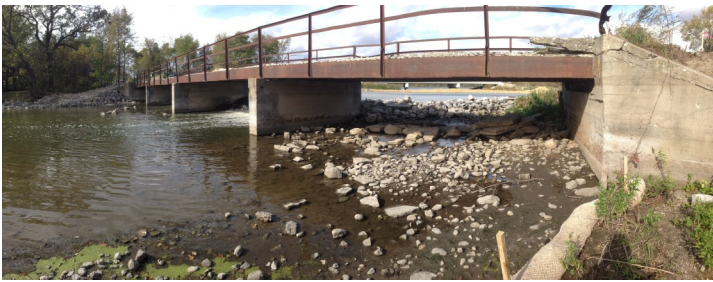
Left: The old, failing dam.
